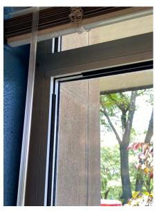
The aluminum and single pane glazing is original to the building and requires replacement as the glazing compound (asbestos containing) and perimeter caulking (asbestos containing) are failing and for improved thermal / energy efficiency. All of these windows are under contract to be replaced this fall (2021) and therefore the costs are excluded from this report.
